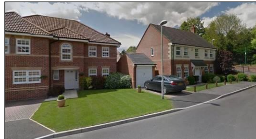
Figure 7.9 New housing off Deadmans Lane
