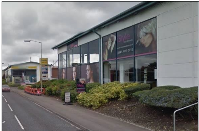
Figure 7.11 Hairdressing salon on Hambridge Road Business Park
