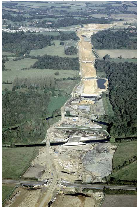
Figure 1.2: Newbury Bypass construction
